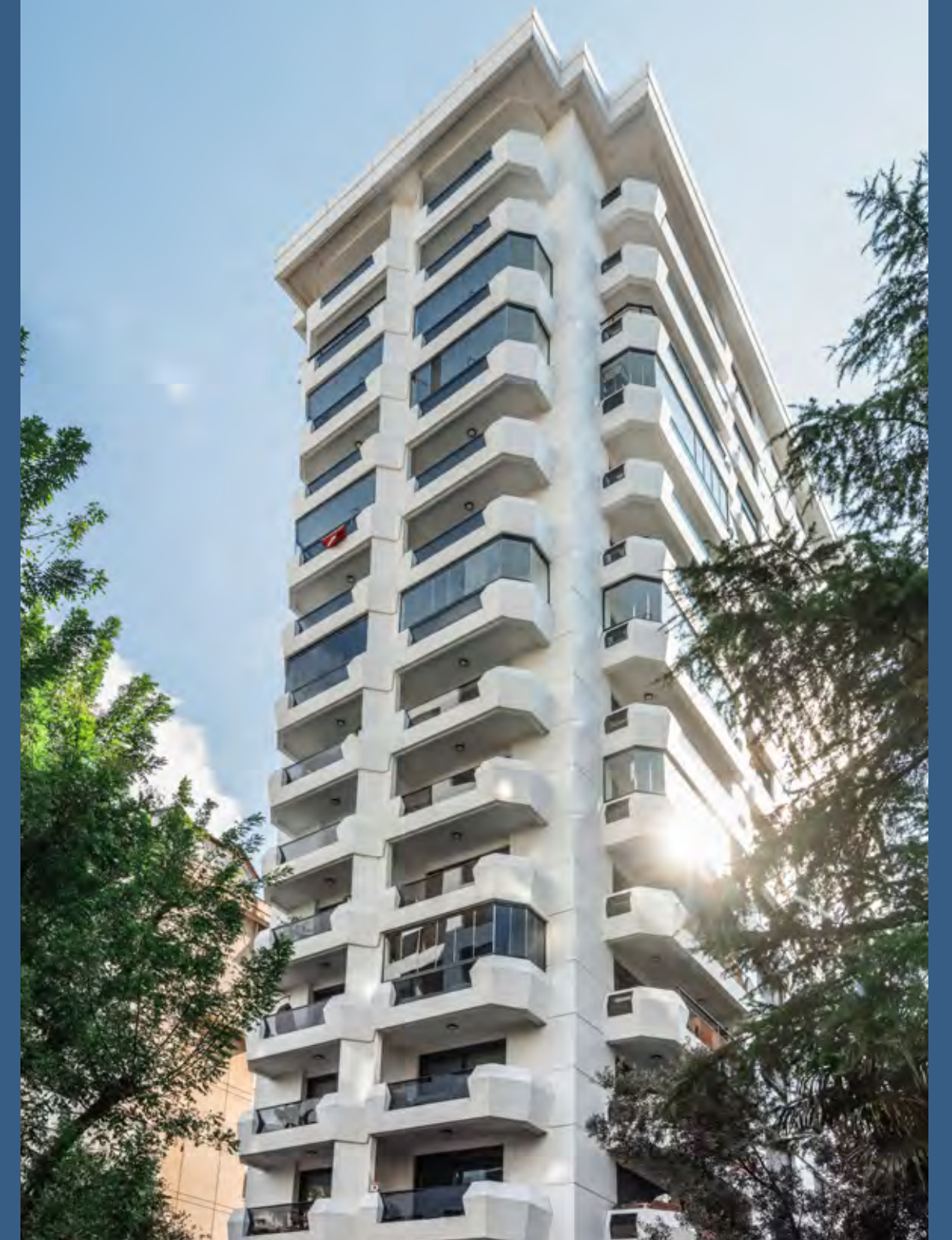
SARAY İNŞAAT Fenerbahçe, İstanbul
