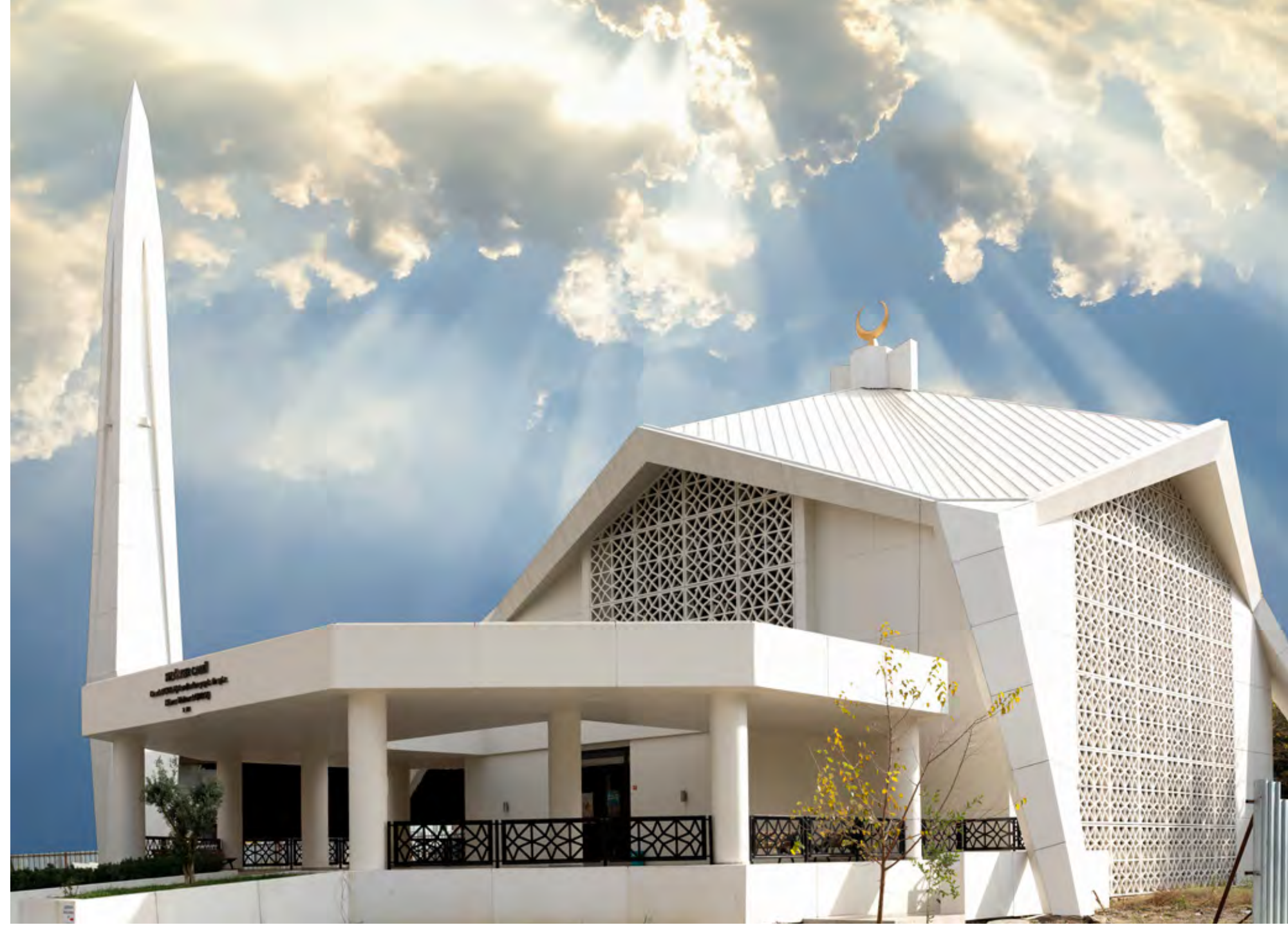
ATAŞEHİR CAMİ Ataşehir Mosque Ataşehir, İstanbul
