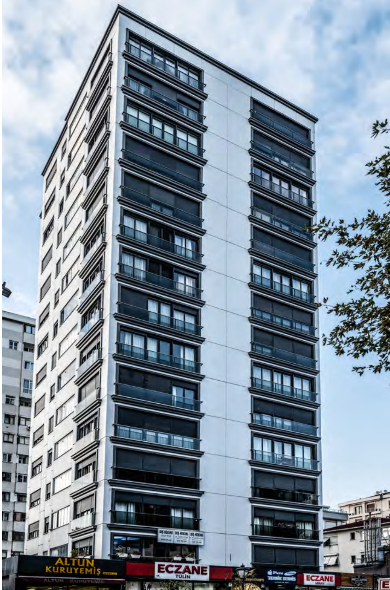
TRC İNŞAAT Erenköy, Kadıköy İstanbul
